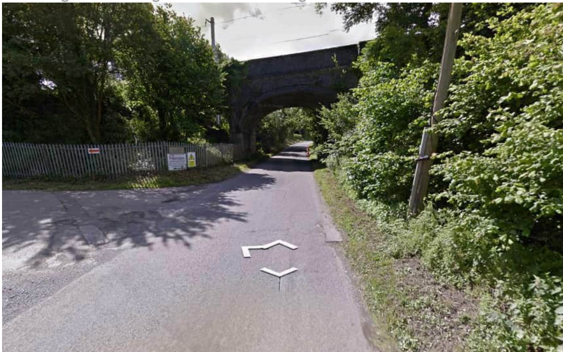
Fosse Way rail bridge (restrictions unknown)
